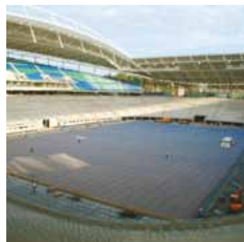
Undersoil pitch heating
