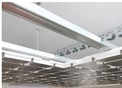
Installation of metal structure with 300 mm pitch
