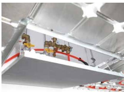
Installation of zone inspection trapdoors where the distribution manifolds are installed
